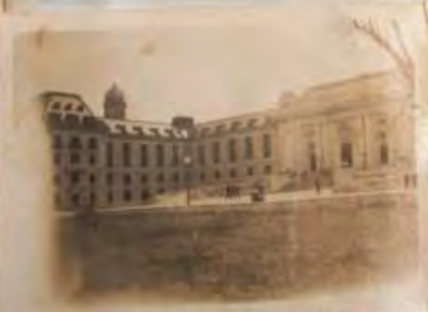
Bancroft Hall Amapolis
