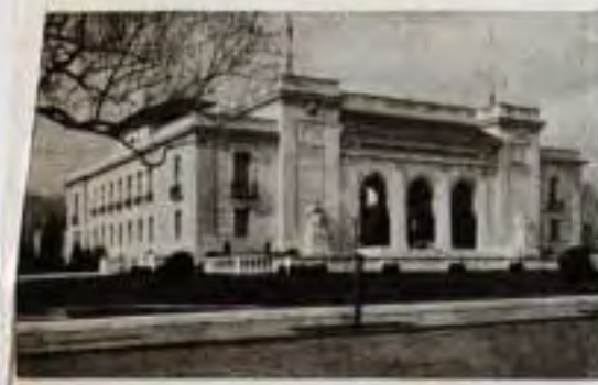
FRONT FACADE OVERLOOKING WHITE HOUSE PARK AND SOUTH SIDE OVERLOOKING POTOMAC PARK
