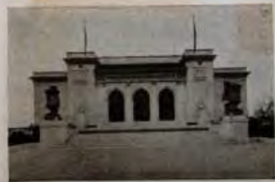
FRONT OR EAST FACADE
